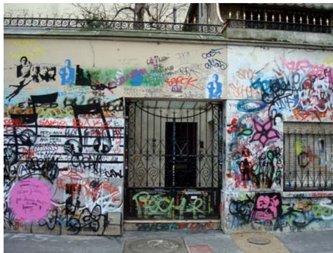
Figure 4. Ubiquitous takeover of (previous) blank wall on city street with ‘graffiti’
